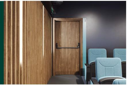
Acoustic rating Rw=42 dB Fire-resistance EI 30 Smoke control
