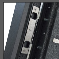
Hinge and anti-burglary bolt socket of the TERMO ALU 84 door frame
